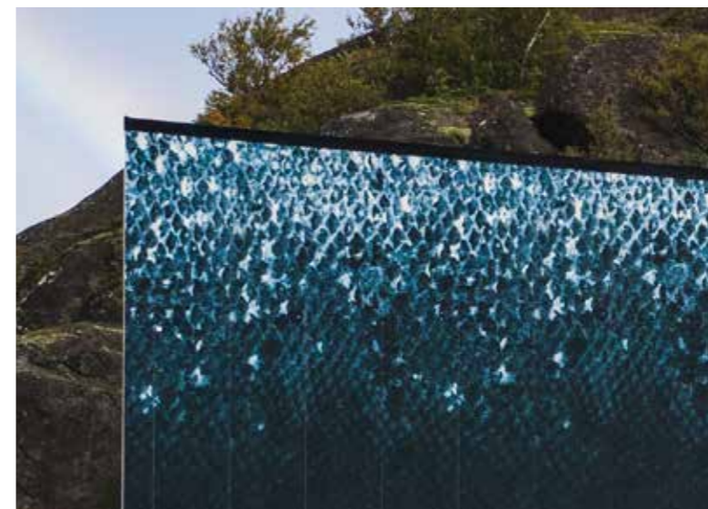
The print patterns on the façade panels create an illusion of salmon scales.
